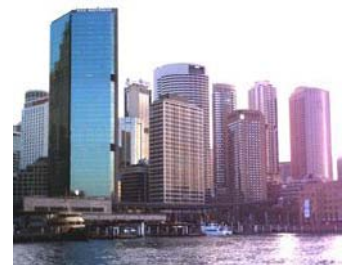
Hermetically sealed buildings in City of Sydney (viewed from Darling Harbour)
